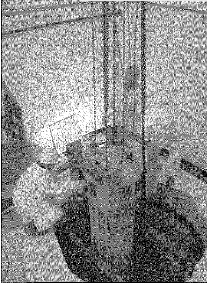
Removing the reactor vessel.
