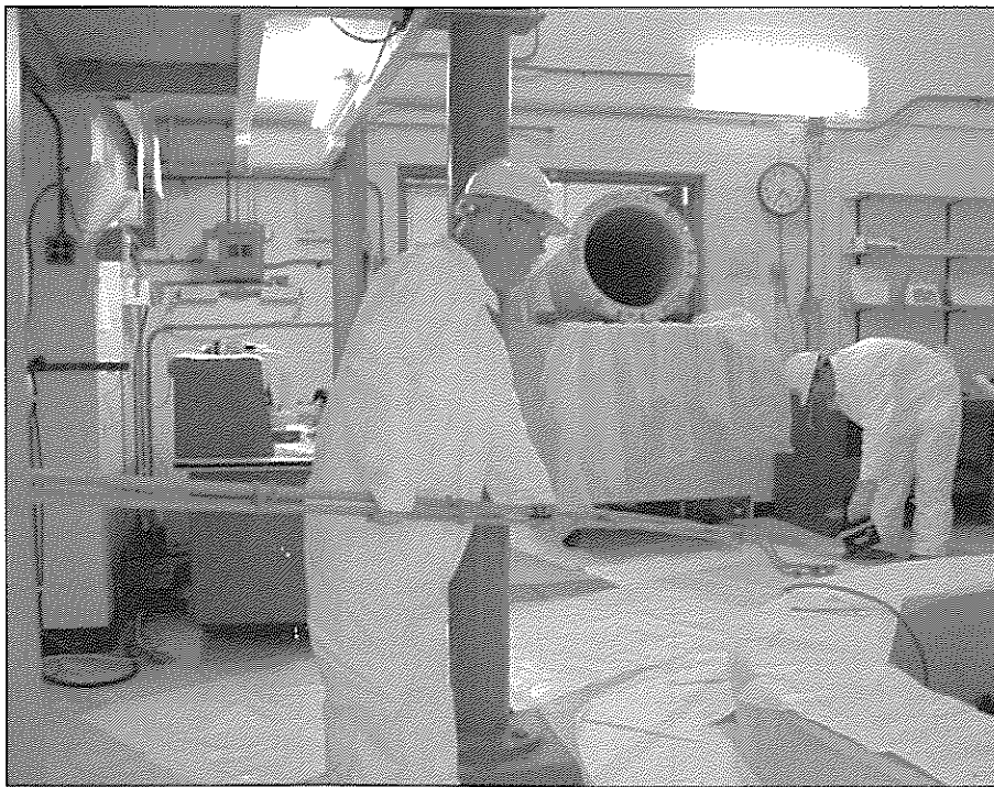
Packing the irradiation tubes.
