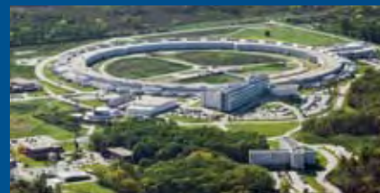
Aerial view of the Advanced Photon Source at Argonne National Laboratory Photo courtesy of Argonne National Laboratory
