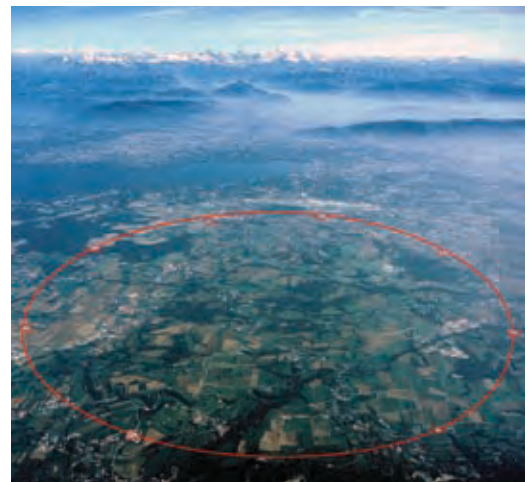
The Large Hadron Collider at CERN, in Geneva, Switzerland Photo courtesy of CERN
