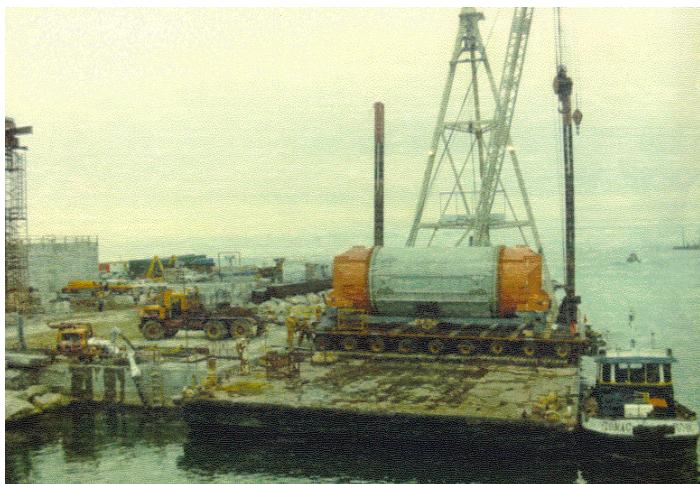
Figure 5.8: Darlington Barge Dock – unloading a 350 tonne generator stator
