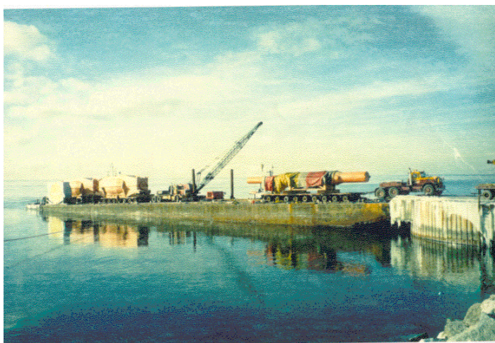
Figure 5.10: Blue Circle dock with barge unloading a 200 tonne generator rotor
