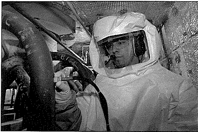
A worker from OPG's Inspection and Maintenance Services, takes precise measurements of a feeder tube inside Unit 1 feeder cabinets. Tight spaces and radiation protection requirements make the task especially challenging. Photo courtesy of Ontario Power Generation
