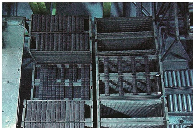
Figure 2: Storage Trays in Spent Fuel Bay.
