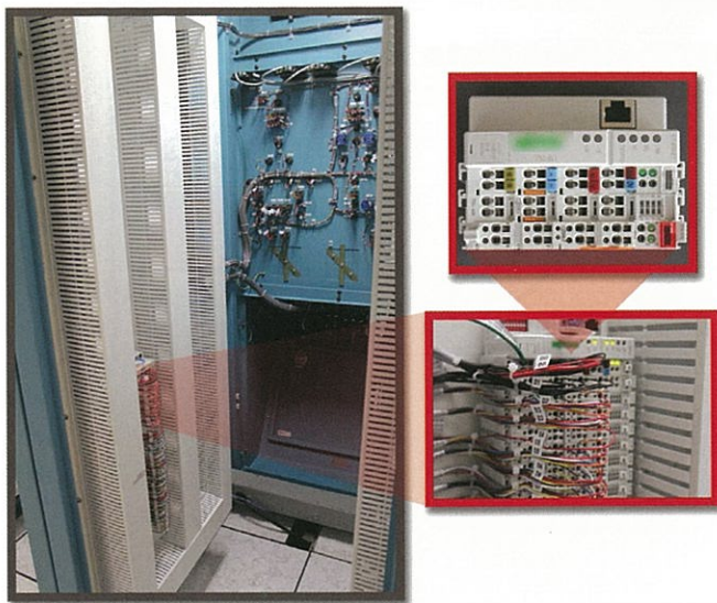
Figure 7: Embalse distributed I/O hardware solution.
