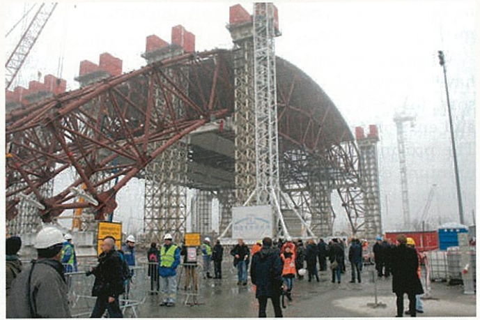
The first arch of the Chernobyl NSC has been raised off the ground (Image: WNN)
