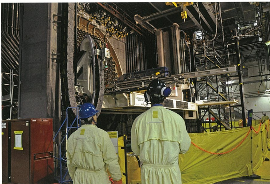
Early refurbishment work at Bruce A showing the reactor face. Photo courtesy of Bruce Power.
