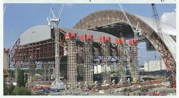
Nearly finished, the second section is lifted in front of the first, more complete section. (Image: Chernobyl NPP)
